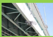
Hanging drone to steel girder
